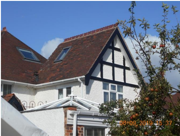
Image 3: First floor extension. (Tudor Cladding, roof alterations, first floor window & the side extension window)
